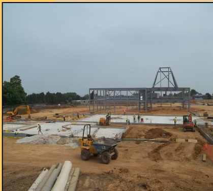
Work being carried out for the preparation of main slab
