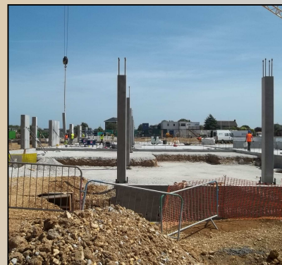
Start of the pre cast panel erection
